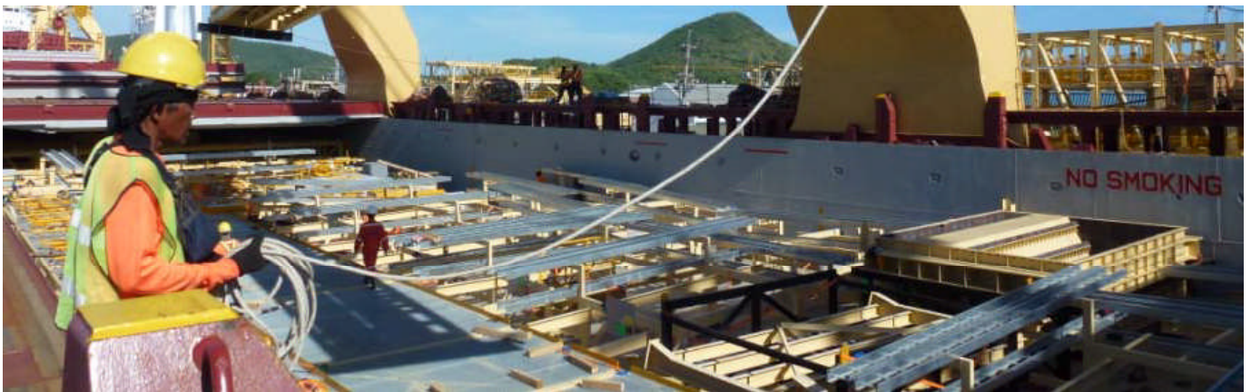
Upon completion of the loading at the tank top and the tween-deck the hatch covers, each with a weight of 51 tons were closed by the ships crew before the start was made to load the deck cargo
